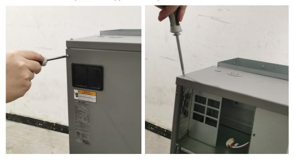
2. Disassemble the electrical box
