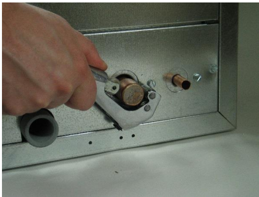
Figure 21. Cut end of connection as shown.
