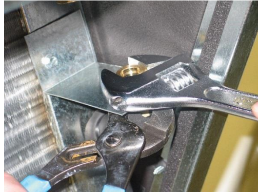
Figure 22. Remove Nut
