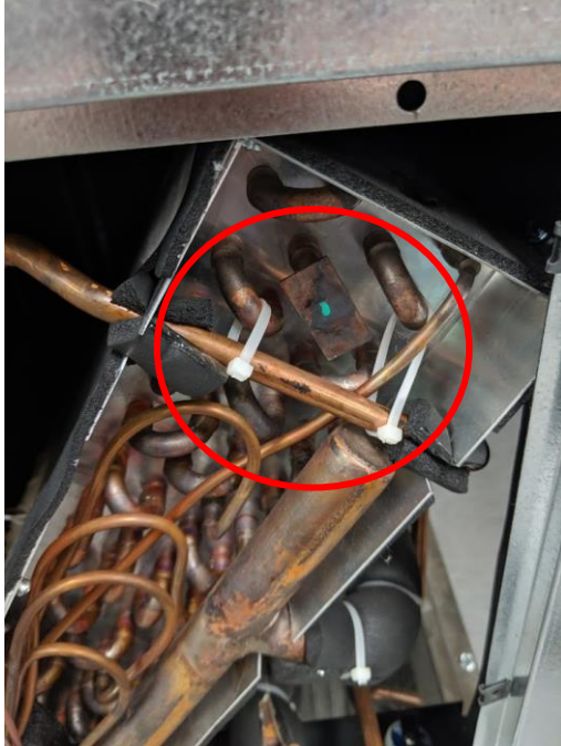
Figure 23. Cut zip ties before installing TXV
